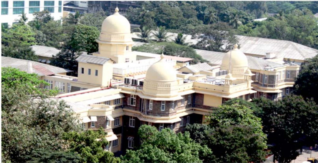
Aerial View of BJWHC.
